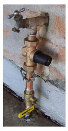
A water pressure regulator is recommended when water pressure is more than 80psi. It holds the pressure below a preset level to make it less likely that high water pressure spikes could cause water to faucet supply lines and appliances to leak. Pressure regulators are an inexpensive insurance against possible expensive water damage.
